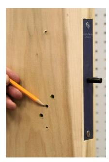
Once all holes and pilot holes have been drilled, enlarge per the mortise lock specifications. In this example the spindle hole is being enlarged from the 1/4" pilot hole to the required 1-1/8" size. Drill all other holes in the same manner.
