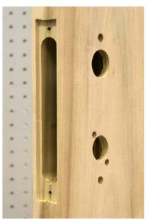
Completed installation, install mortise lock per factory instructions.
