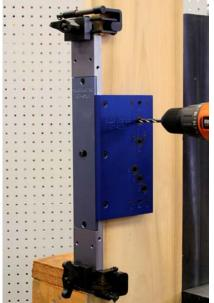
Working from one side of the door, drill all holes that are required for the lock function you are using. Drill holes that go through the door only half way. The back of this manual will identify hole locations and sizes. All large holes will be piloted with a 1/4" drill bit and enlarged with a hole saw once the clamp is removed.
