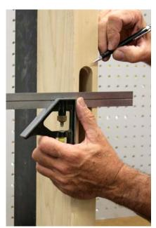
To center the template we must find the center of the lock mortise. Using a combination square, make a pencil line at the top and bottom of the mortise as shown.
