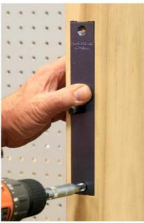
The second half of the template will attach to the faceplate area. Use a self centering drill to locate the screw holes required by the mortise lock. This will help with alignment and prevent binds when the lock is installed. Use the factory supplied screws to attach to the door.
